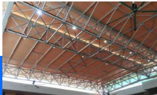
Kalyani School Sports Courtyard, Pune
