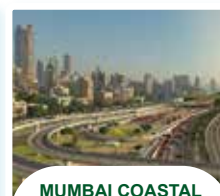
MUMBAI COASTAL ROAD MEGA PROJECT
