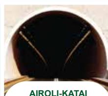
AIROLI-KATAI NAKA TUNNEL
