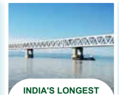
INDIA'S LONGEST BOGIBEEL BRIDGE
