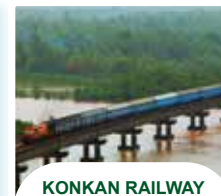
KONKAN RAILWAY PROJECT
