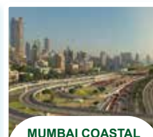
MUMBAI COASTAL ROAD MEGA PROJECT
