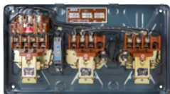
Interior View of MK2 FASD
