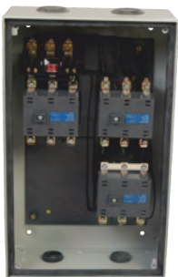
Interior View of ML SASD
