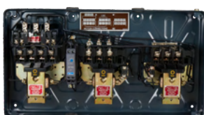
Interior View of MK1 FASD
