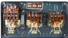
Interior View of MK2 FASD
