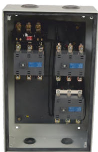
Interior View of ML SASD
